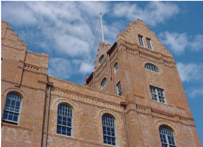
YBOR BREWERY RESTORATION
